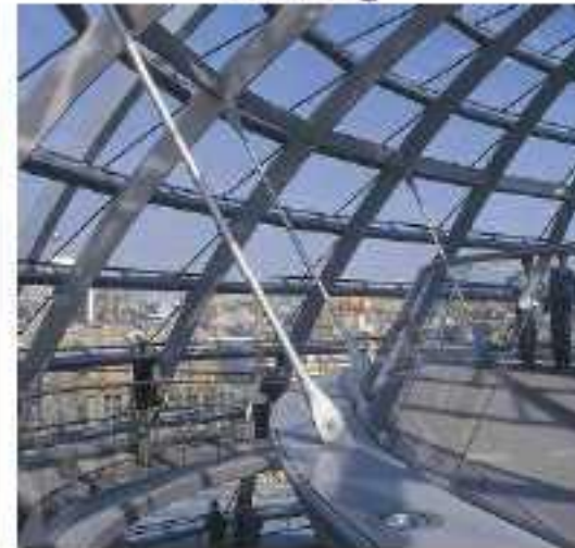
Roof & Overhead Glazing
