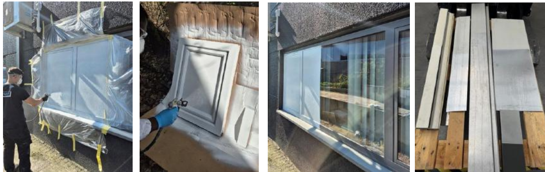
Applied by airless spray equipment on glass, aluminium, pvc
